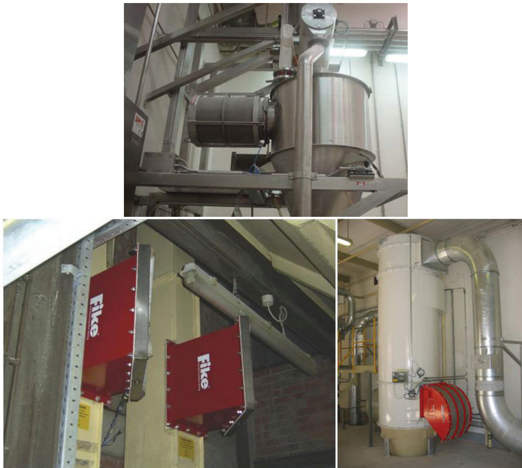
Figure 4: Fike FlamQuench IITM flameless venting device on a hopper (cylindrical), on a bucket elevator and on a filter installation (square)
