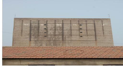
Figure 2: The layout of Hongjin tile factory chimney (north-south)
