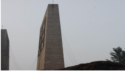
Figure 1: Hongjin tile factory plate wet exhaust chimney map (east-west)
