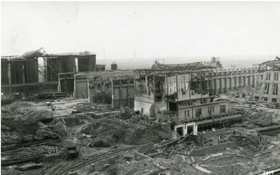
Figure 2: Destruction in the neighbourhood of the exploded silo
