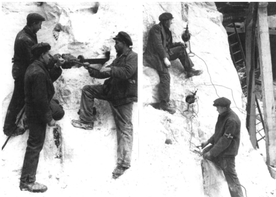
Figure 3: Preparation of blasting operation
