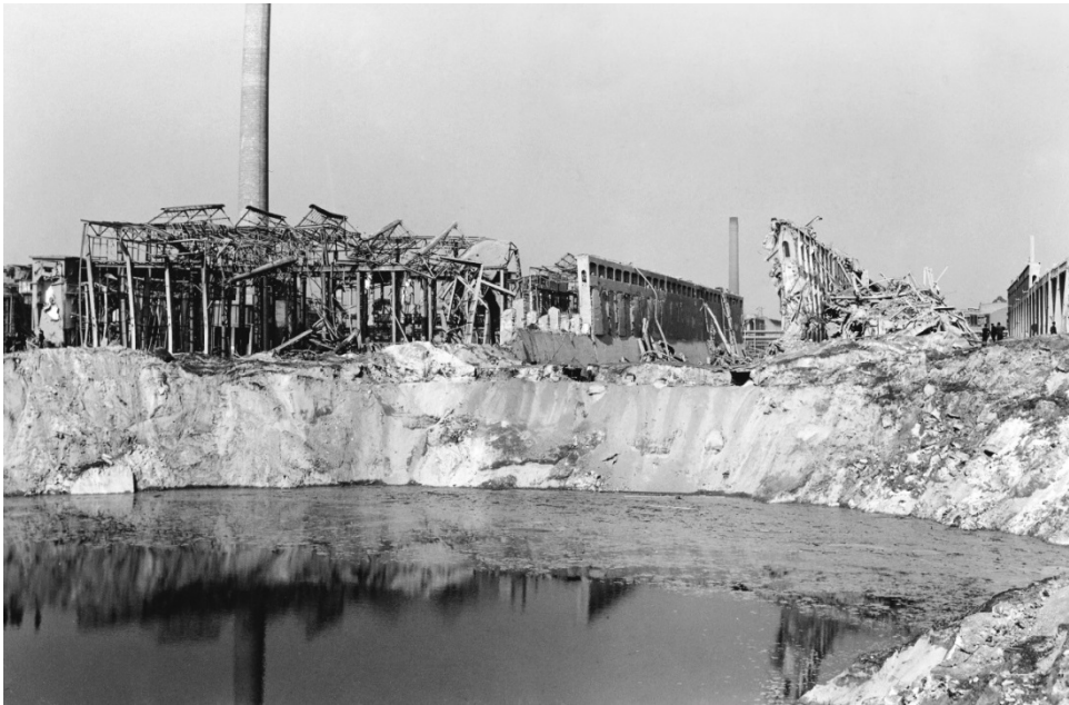
Figure 1: View of the explosion crater
