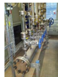
Figure 11 Venturi nozzle metering section
