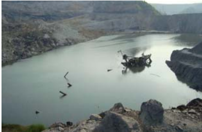
Figure 1: Regional Failure of benches at Umrer OCP, M/s WCL
