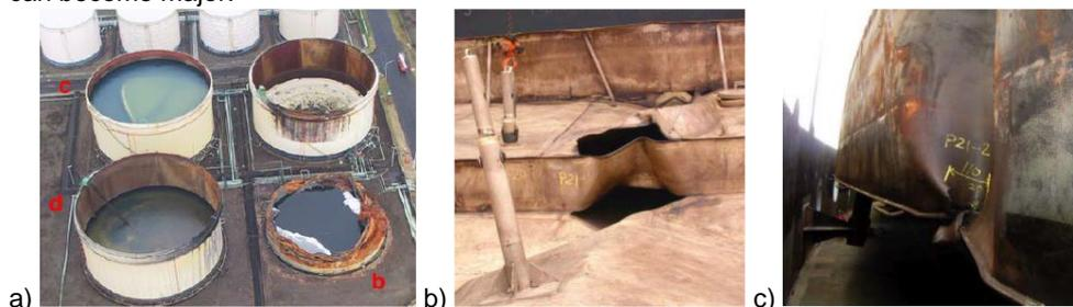
Figure 1: a) tilting of floating roof and burned tank (Hatayama, 2008), b) buckling of inner pontoon, c) buckling of outer pontoon (Yamauchi et al., 2006)
