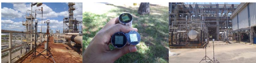
Figure 1: Ground measurement station and monitoring sensors
