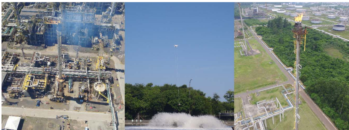
Figure 2: Unmanned air vehicle (quadricopter drone) used to take the monitoring sensors close to stack SRU, aerated lagoon and Flare
