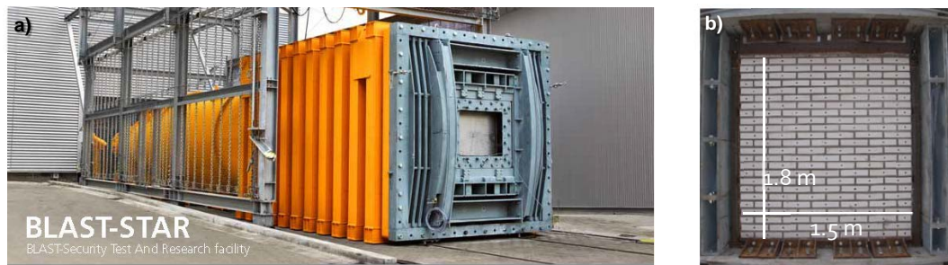
Figure 1: a): Shock tube at the Fraunhofer Institute for High-Speed Dynamics. b): Masonry wall specimen, at the end of the shock tube. Black markers on the brick faces are used for feature detection and automatic particle tracking.
