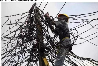
Figure 1: Sample of a distribution line that are not properly maintained
