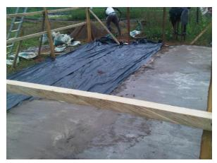
Figure 1: The Greenhouse floor at the DPC level
