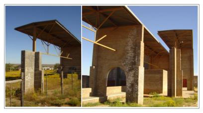
Figure 9: No maintenance on the cement brick-constructed Steinkopf Community Centre in the Northern Cape Province, South Africa
