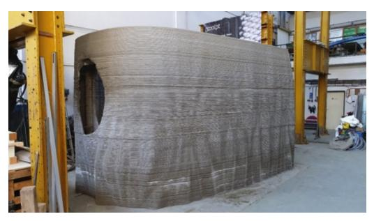
FIGURE 6. Printed segment of the PRVOK.
