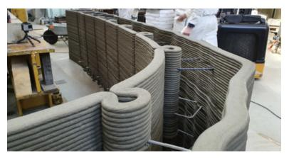
FIGURE 7. Construction of the wall during the printing.
