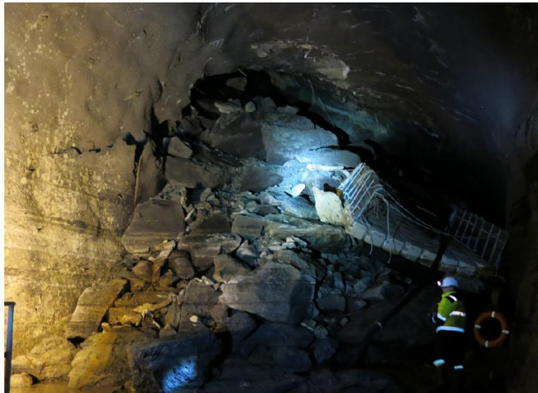
FIGURE 3. The collapse 1 after water pumping completion.
