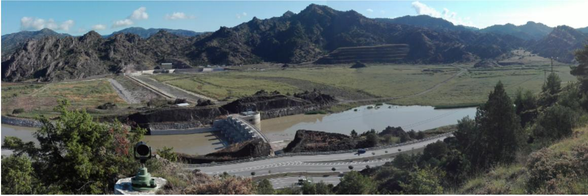
FIGURE 1. Discharged dam with the inlet structures and mountain range crossed by the headrace tunnel.
