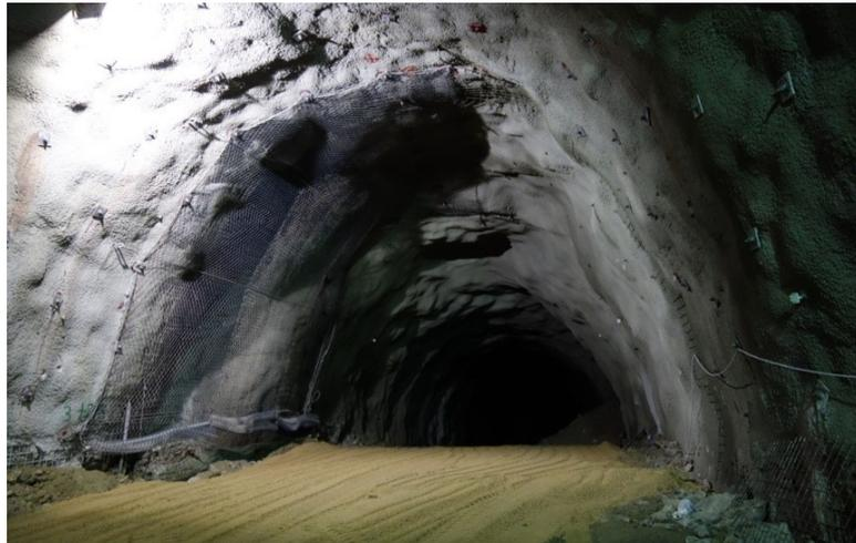
FIGURE 4. The collapse 2 mouth protection by the high-tensile steel mesh.
