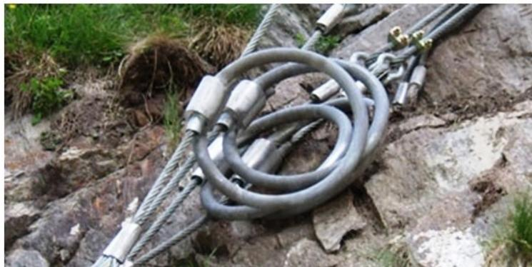
FIGURE 7. Detail of a loop-type breaking element (energy absorber) of the dynamic barrier.
