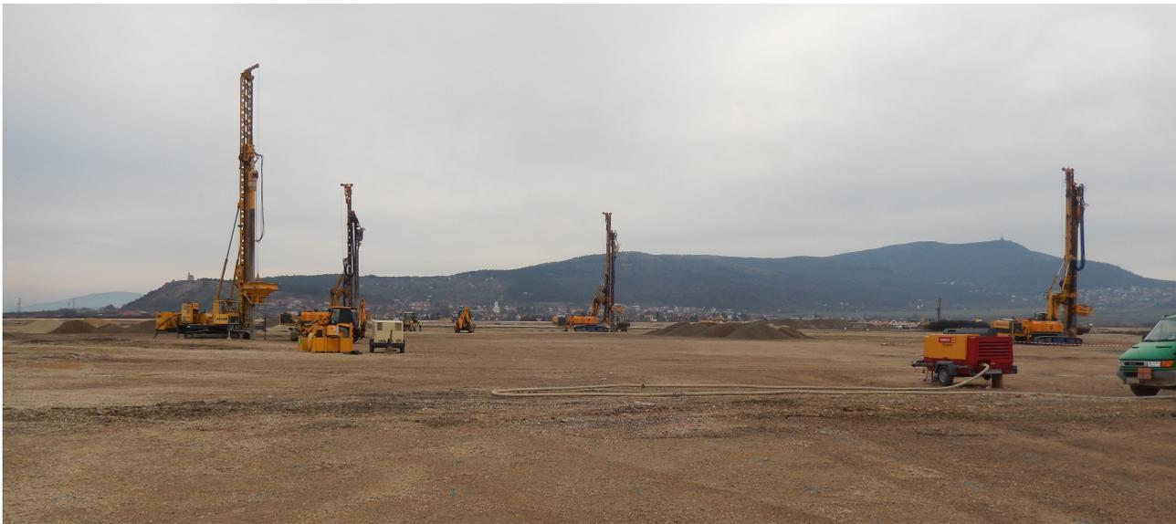
FIGURE 2. Overall view on making stone columns.
