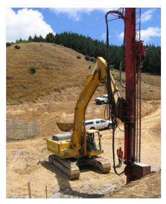
FIGURE 4. Vertical lime-cement columns – technology COLMIX [3].
