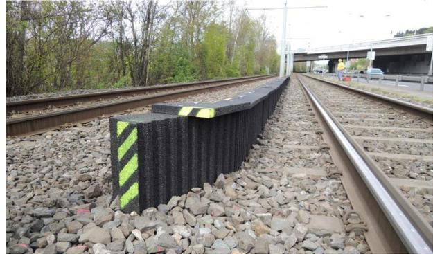
FIGURE 10. Municipal Noise-absorbing Screen after modification.
