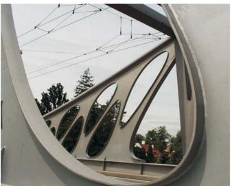
Fig. 10: Long Bridge in České Budějovice. Built 1999 by Roman Koucký and Tomáš Rotter. The structure of the bridge (left). The rubber-like deformed openings of the side beams (right). (Authors of figures: Lenka Popelová and the database of the VCPD, **CTU** in **Prague.**)
