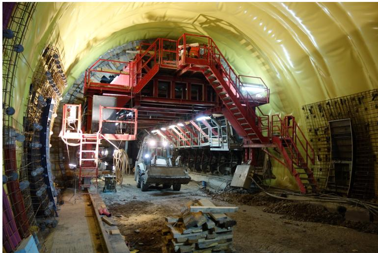
FIGURE 2. The secondary lining construction from in situ cast concrete (photo Hilar).
