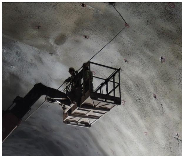
FIGURE 3. Installation of rockbolts (photo Hilar).
