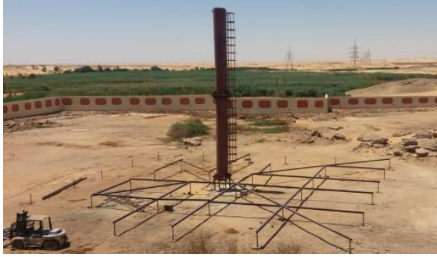
FIGURE 2. Prototype in Aswan (under construction).
