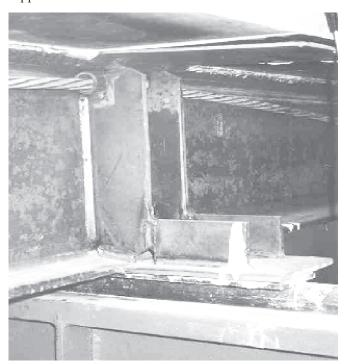
Fig. 2: Structural details at the inner support section
