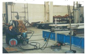
Fig. 3: Stressing of tendons by means of a hydraulic jack unit
