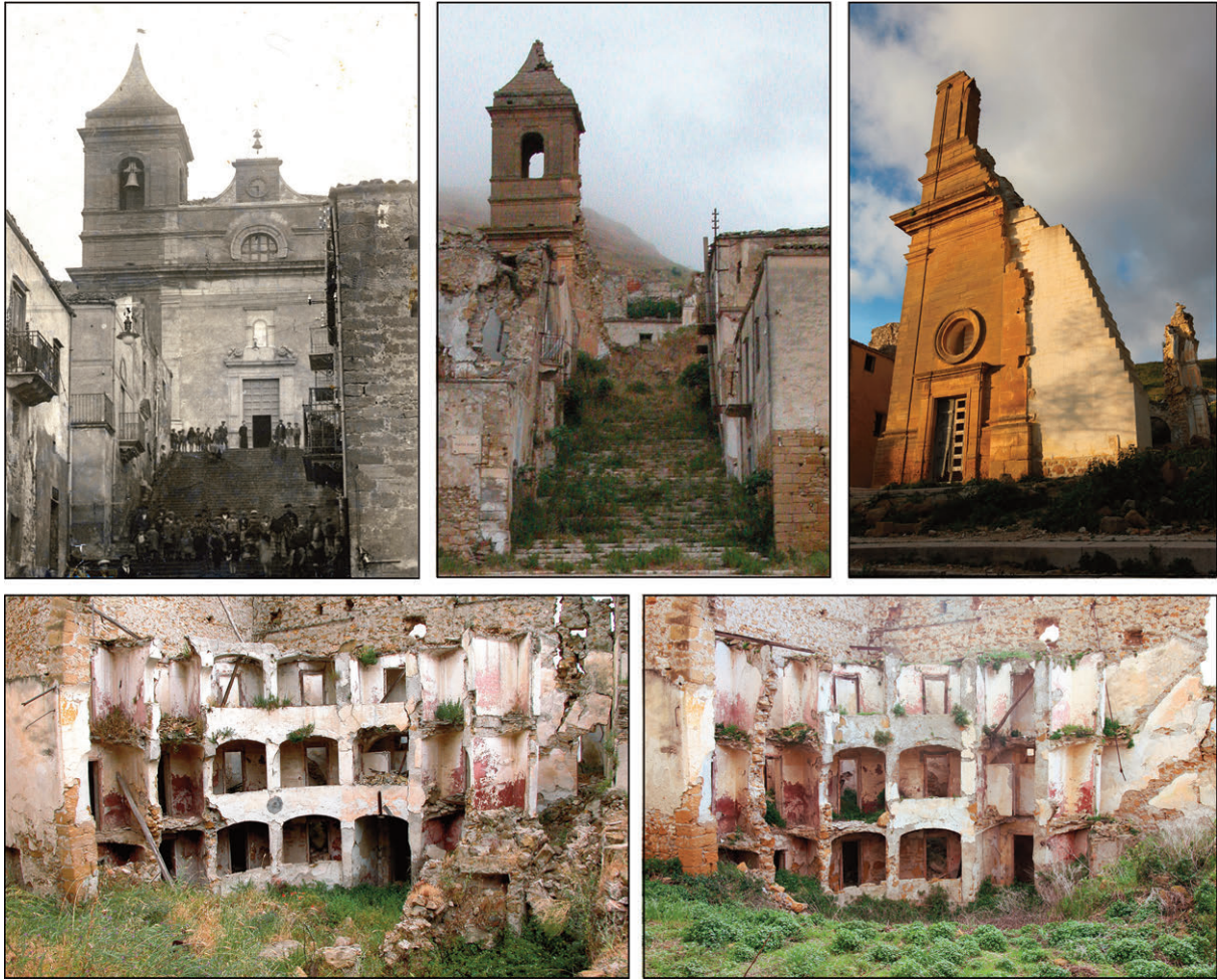
Figure 10. Poggioreale, the symbolic places disappearing: (top) the bell tower of the Holy Mother church in the early 1900s (courtesy of G. Coco), in 2003 and finally as it appears today, after the collapse occurring in 2009. (bottom) the degradation of the small theatre along the main street, is apparent in just 15 years.
