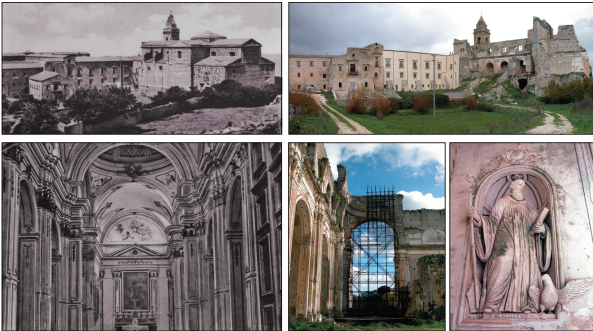
Figure 11. Santa Maria del bosco: (top) the abbey in the mid-1900s (courtesy of Mons. F. Ferina) and the present-day condition. Note the dramatic difference between the part of monastery entirely restored (privately owned, now it is a resort) while the church is collapsing. (bottom) the inner of the church in the mid-1900s, now the remains of apse, nave and ornaments are without any protection, exposed to very fast degradation processes.
