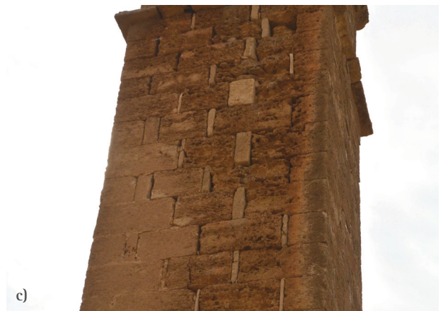
FIGURE 5. Space between the blocks has been filled with stone slabs.
