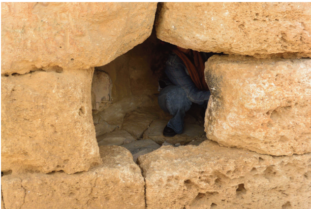
FIGURE 4. Small chamber at the basement.
