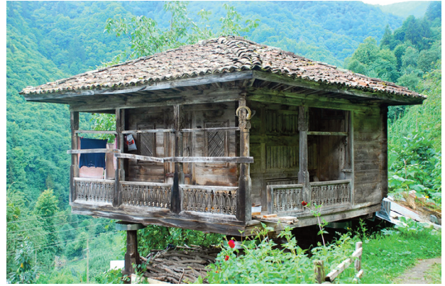
FIGURE 21. A block timber grain warehouse in Rize (Photo: Dışkaya, N.).
