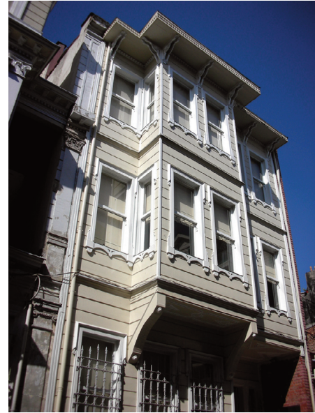
FIGURE 40. A 19 th Century timber building in Istanbul (Photo: Dışkaya, H.).
