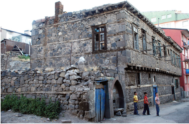
FIGURE 41. Rubble stone house with timber lacing, Erzurum, (Photo: Dışkaya, N.).
