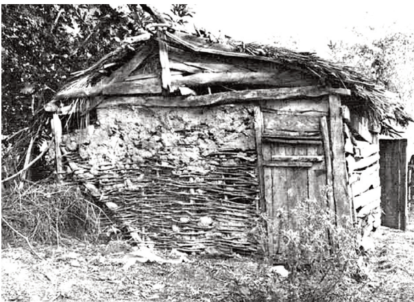
FIGURE 17. Interlaced twigs on a timber skeleton rural building [Yakar, J. et al.].
