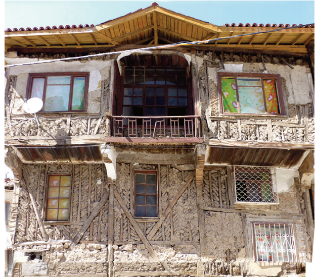
FIGURE 30. A sample building for herringbone infill style in Amasya (Photo: Dışkaya, N.).
