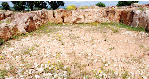
FIGURE 10. Section view of a Hittite foundation in Šapinuva B.C. 1500 (Photo: Dışkaya, N.).
