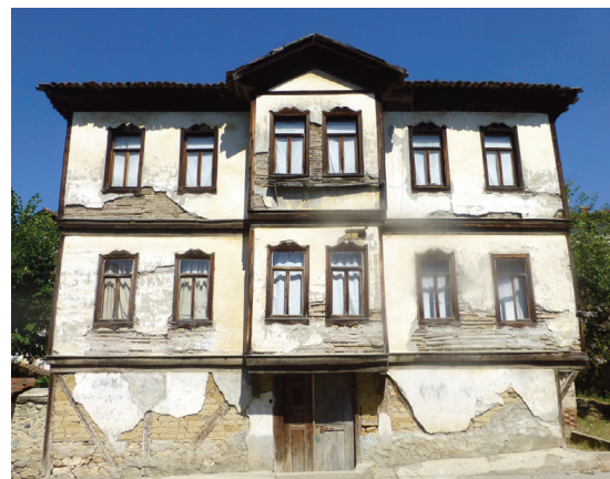
FIGURE 34. Baghdadi plastered timber building in Boyabat (Photo: Dışkaya, H.).
