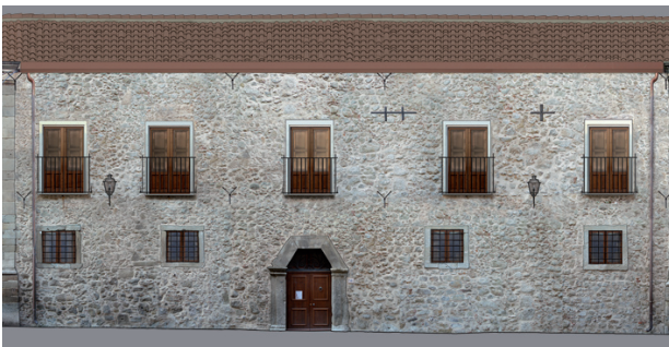
FIGURE 6. Ficarra, Busacca Palace, the buttresses at the edges.
