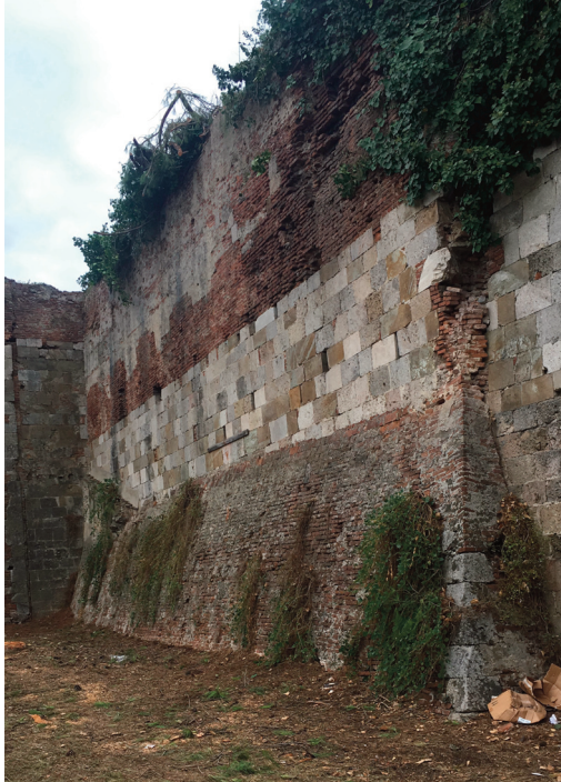
FIGURE 5. Pisa, buttress to contain the falling over of a part of city wall.
