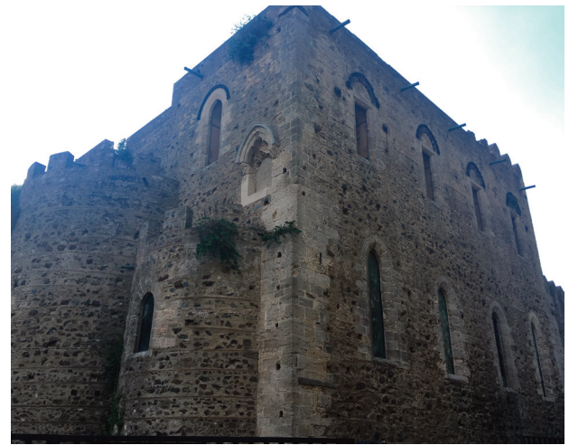
FIGURE 2. Messina, Santa Maria della Valle: wall with red brick layers from the Norman period.
