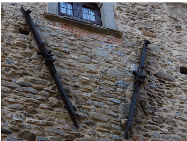
FIGURE 19. Iron chains inserted in the external stonework of the Vicari Palace in Scarperia (FI).
