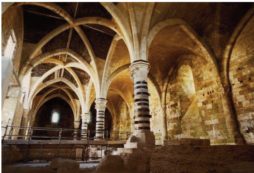
FIGURE 15. Siracuse, Maniace Castle, note how veils were made respecting the physical-mechanical characteristics of the materials used.
