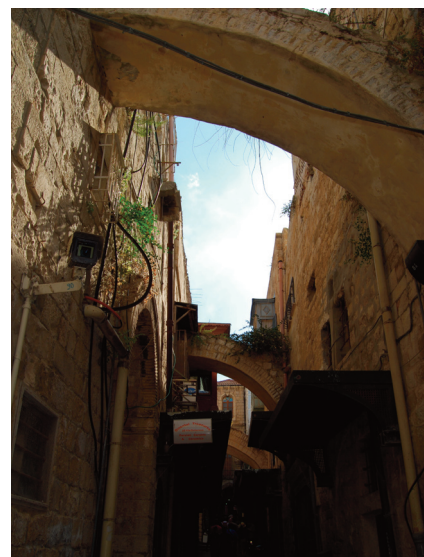
FIGURE 10. Jerusalem, Rampant arches to counteract the vault thrust.
