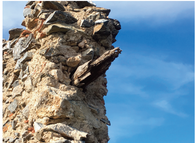
FIGURE 11. Gioiosa Guardia (Me), lodging for wooden beams drowned in the masonry.
