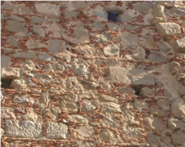
FIGURE 14. Ficarra (Me), masonry palimpsest with earthenware used to fill lesions.
