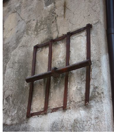
FIGURE 8. Roggiano Gravina (Cz), anchor-plates.
