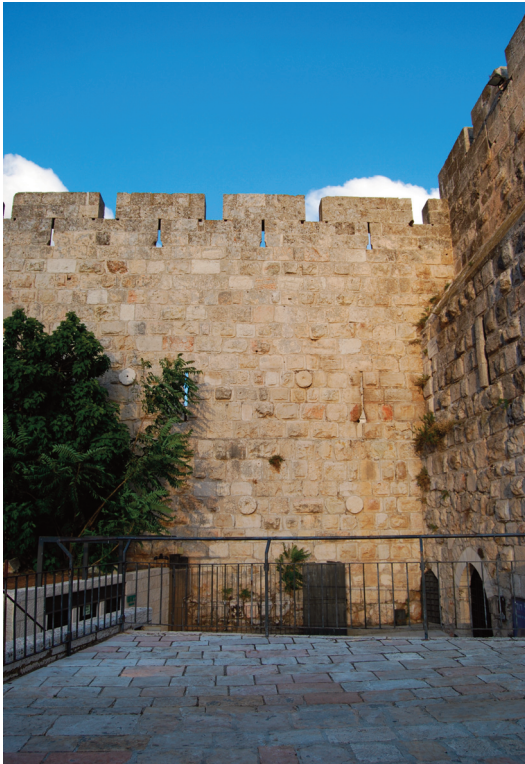
FIGURE 3. Jerusalem, binding stones created with re-used column drums.
