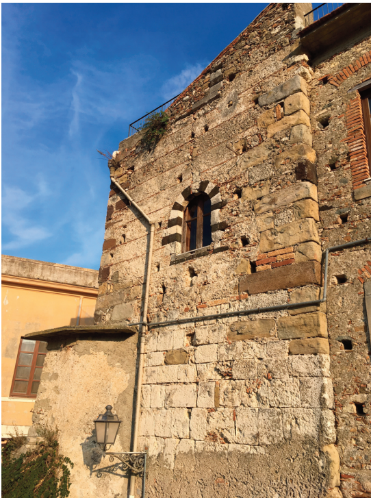
FIGURE 1. Patti (Me), close to the Cathedral: wall with brick layers from the Norman period.
