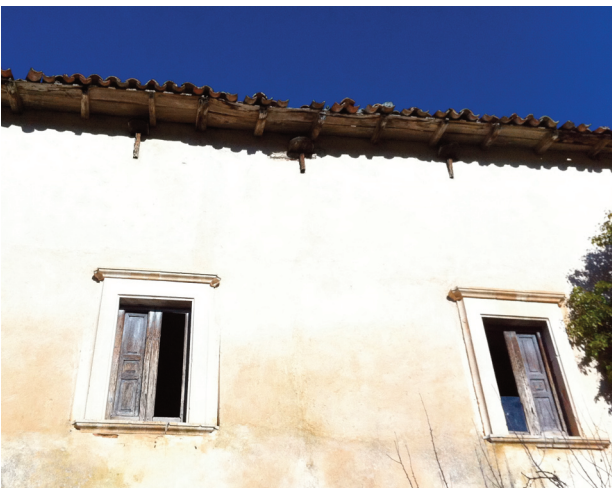
FIGURE 7. San Pio (Aq), wooden chain and anchor-plate.
