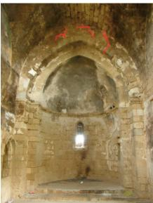
FIGURE 8. Deteriorated state of (a) the vaulted roof and of (b) the internal double–arch (with highlighted cracks at the top).
