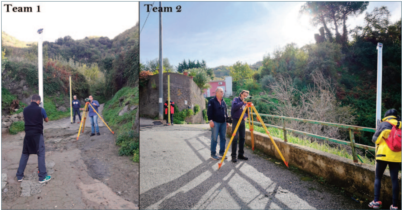
FIGURE 5. Field measurements in the leveling survey.
