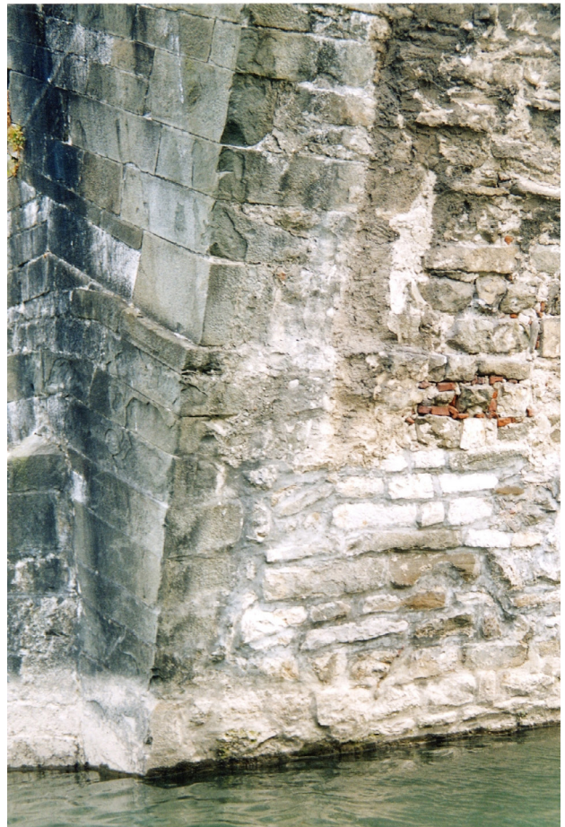
Figure 3. Detail of the masonry texture on the main arch: at the left haunch on the downstream side (top) and at the left springer on the upstream side (bottom).
