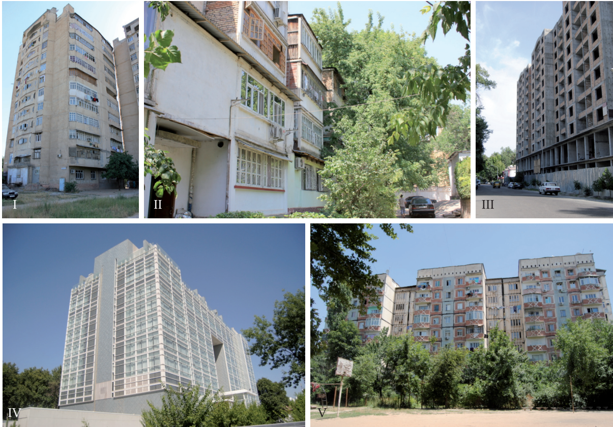
Figure 2. Photos of the 5 buildings in Dushanbe where ambient vibration measurements were performed. (I) 12 story monolithic RC building, (II) 4 story confined masonry building, (III) 12 story RC dual system building under construction, (IV) Serena Hotel and (V) 9 story reinforced large panel precast concrete building.
