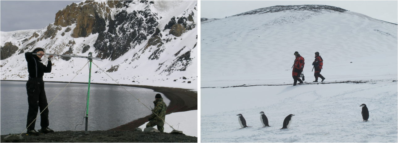
Figure 3. Maintenance operations of a seismic network station during the 2003-2004 survey. Left: inspection of the radio telemetry antenna; right: battery replacement.
