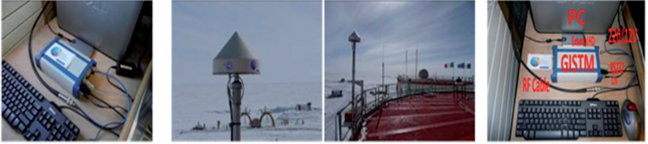
Figure 3. The ISACCO-DMC0 station installation (latitude, 75.1001°S; longitude, 123.333°E, 3280 m a.s.l.).
