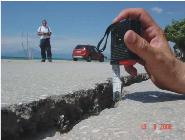
Figure 9. Structural damages at the waterfront area of the village Vrahneika. Examples of failures on pavement with both throw and opening components (left: throw = 3 cm and opening = 2 cm; right: opening = 4 cm).
