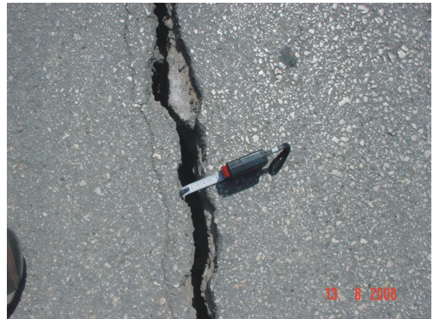
Figure 9. Structural damages at the waterfront area of the village Vrahneika. Examples of failures on pavement with both throw and opening components (left: throw = 3 cm and opening = 2 cm; right: opening = 4 cm).
