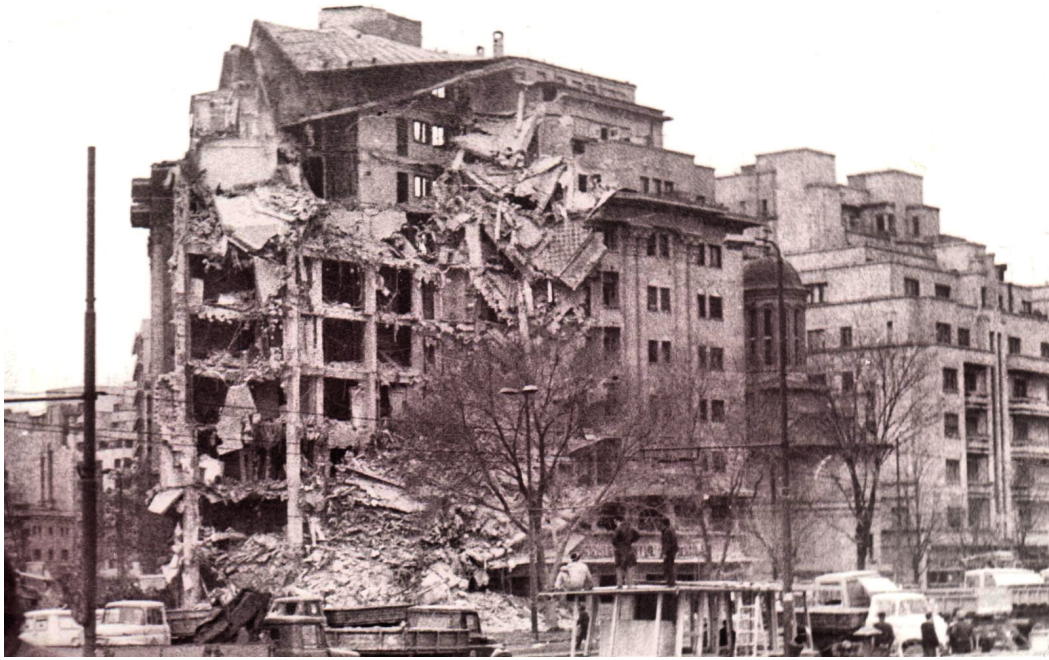
Figure 9. Partial collapse of the 'Dunarea' building (reinforced concrete frame building with masonry infill walls) (photo by Ene [1977]).
