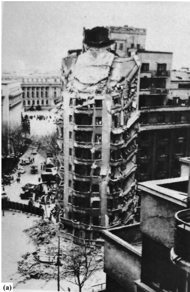
Figure 8. Partial collapse of buildings. (a) The Wilson building (reinforced concrete frame building with masonry infill walls). (b) A masonry building. (photos by Hirosawa [2007]).
