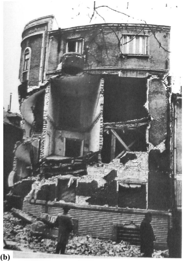
Figure 8. Partial collapse of buildings. (a) The Wilson building (reinforced concrete frame building with masonry infill walls). (b) A masonry building. (photos by Hirosawa [2007]).
