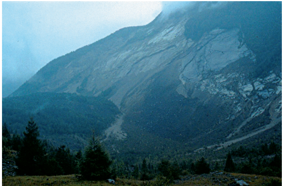
Figure 3. The present rock mass landslide.
