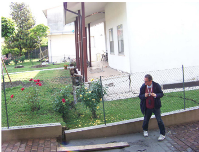
Figure 22. Environmental effects accompanying the May 20, 2012, M_W 5.9, Finale Emilia earthquake. The ground failure associated to sand liquefaction at San Carlo, 30 km ESE of Mirandola. Dorian Castaldini shown for scale. The photograph was taken on May 21, 2012.
