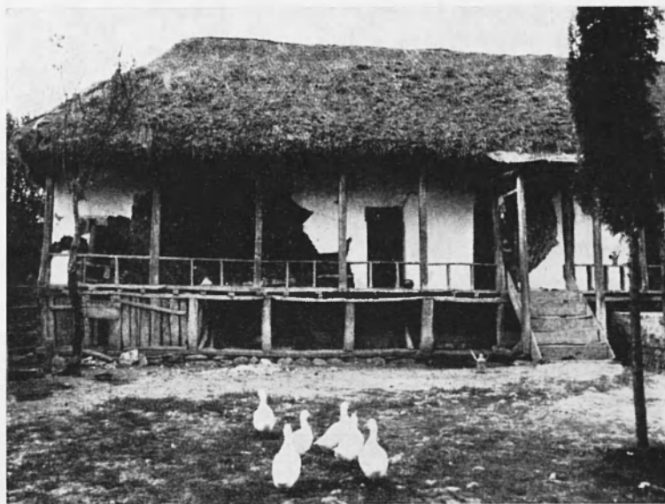
Plate 2 - Local type house in Deraz Kola. All inner and outer walls will have to be rebuilt, but the timber framework and roof will only need minor repairs.
