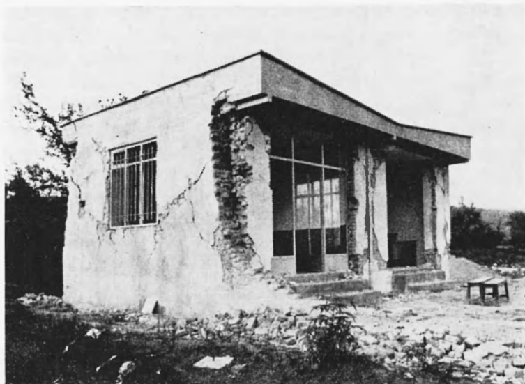
Plate 1 - Shops in Govan Kola. These kiln-brick and mortar constructions generally suffered more than the local type houses.
