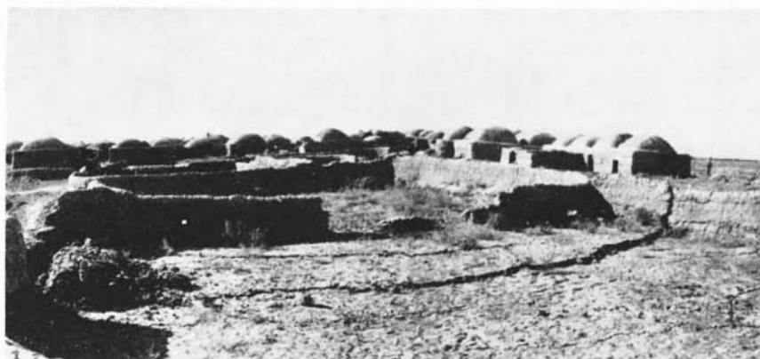
Fig. 14 - Salayani - - View of the easternmost houses of the village (north of Khaki road, see plan, Fig. 11). Lurch fractures in the foreground cross mud walls and houses with only partial collapse of the latter.
