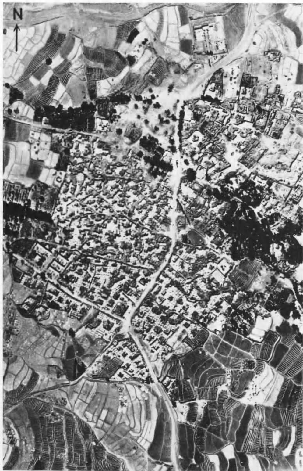
Fig. 8 — Khezri — Aerial photograph taken after the 1968 earthquake. The northern entrance west of the road is being bulldozed. Damage is sporadic throughout the village. At the western edge of the village, Government houses built from kilnbricks are standing undamaged. Note the narrow winding streets and compact structure of housing.
