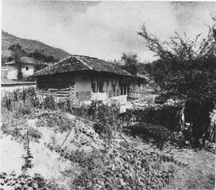
Pl. V - HOUSE IN SANGECHAL -- The large amount of timber used in the walls is an innovation after the 1957 earthquake. The roof is (as in 1957?) of wood shingle. The mound and garden in the left foreground mark the foundations of a house which was destroyed in the 1957 earthquake. 180 people out of a population of about 4000 were killed by the earthquake in Sangechal.
