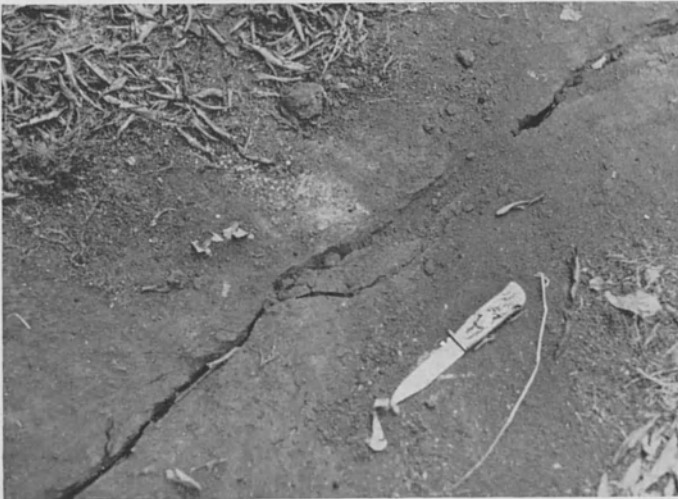
Fig. 4 - A fracture in the ground (Tremestieri, Mt. Etna), with a vertical displacement of 1 cm and a horizontal clockwise one of 1.5 cm, that preceded the Mascalucia earthquake of 23rd August 1980.
