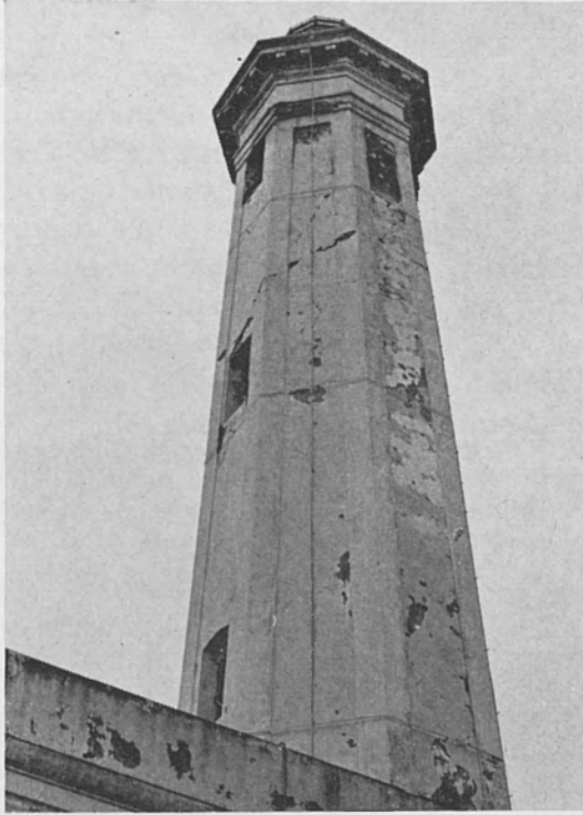
Fig. 3 - The Gelso Lighthouse (the Island of Vulcano, Aeolian Islands) with the tower broken and twisted anticlockwise two-thirds the way up (earthquake of 15 th April 1978).
