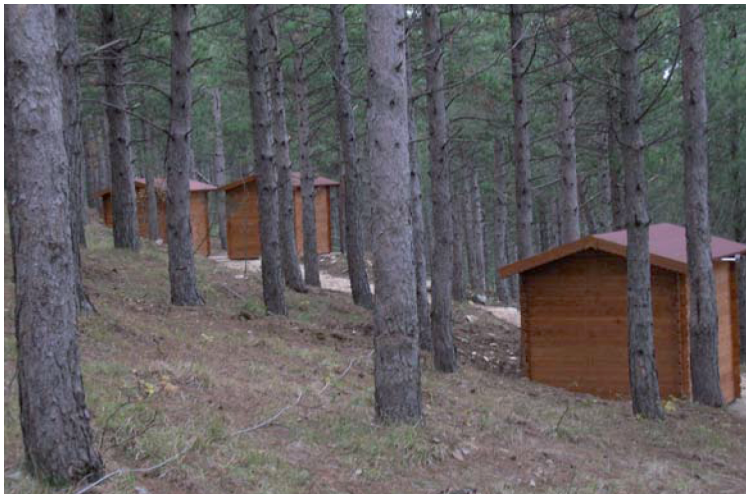
Fig. 3. A view of Durovia station.
