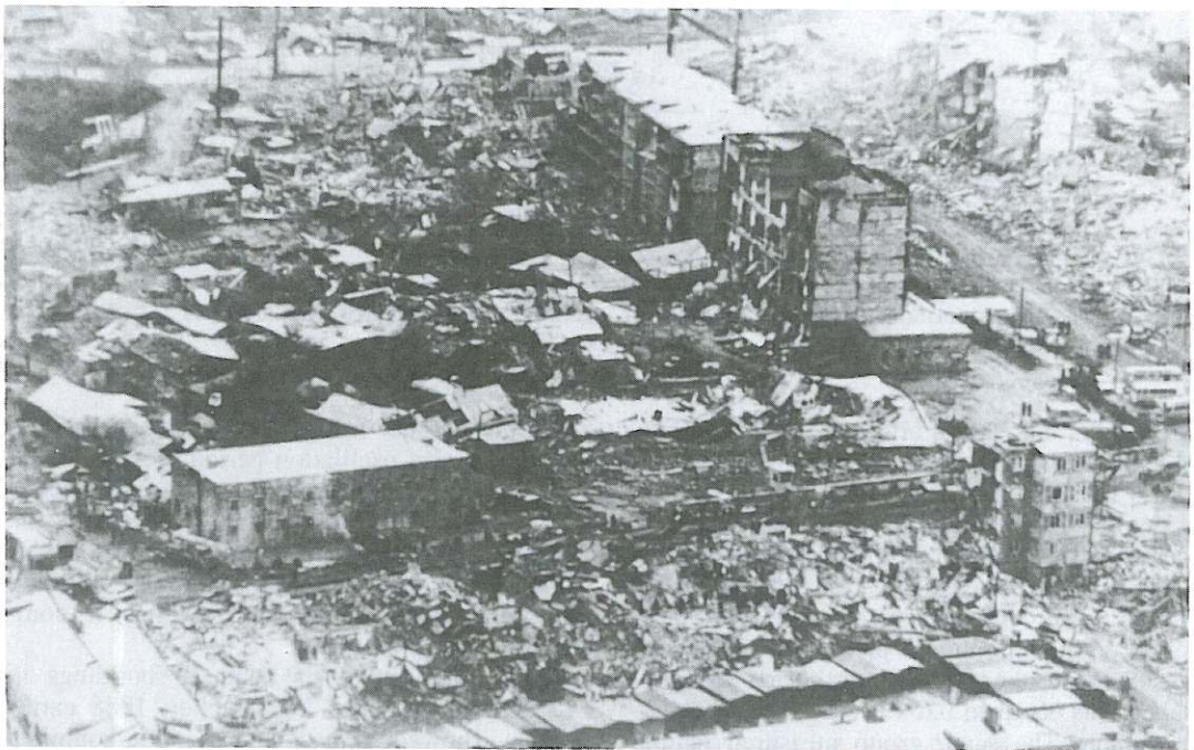
Fig. 27. Destruction in the 10-intensity isoseism zone.
