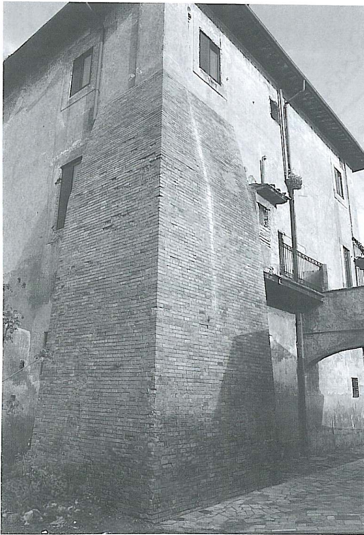
Fig. 4. Reinforcement wall for the damaged edge of the Alberoni Palace.
