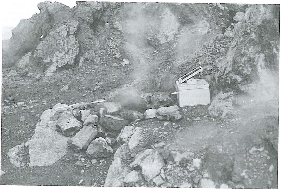
Fig. 1. Photograph of the extensometer installed across a fracture on the summit of Merapi (Java, Indonesia). The box contains a one channel electronic system and the battery. The Argos antenna and the solar panel are fixed on the box. The wire of the extensometer is protected by a plastic tube.
