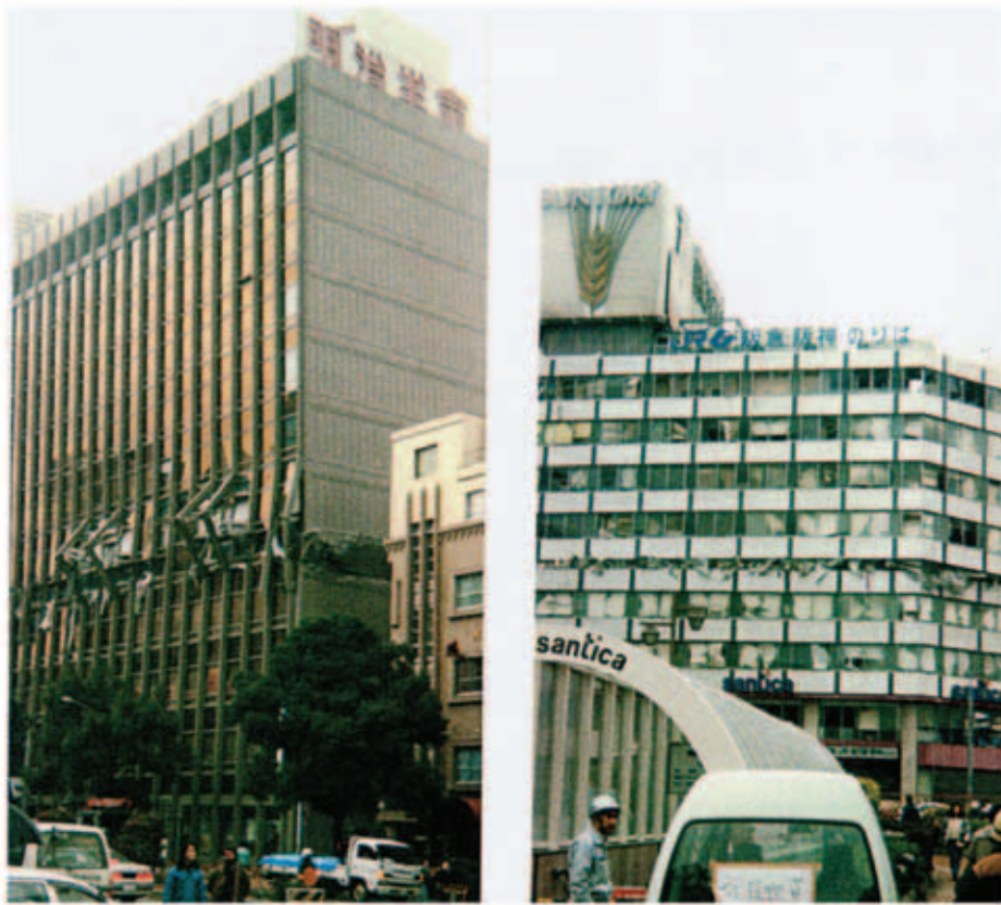
Fig. 1. Story collapse of reinforced concrete frames in Kobe earthquake.
