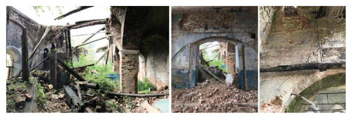
Figure 2. The state of neglect and the lack of conservation present critical situations of widespread instability among the masonry systems, clearly exposing the structure to the damage affecting its elements. Robustness instabilities in the structural complex of the Church of the Transfiguration, Pyskor, defining the increasing frameworks of damage that will destroy these buildings without specific lines of intervention.
