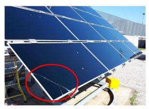
Figure 7. Detail of the broken module in plant  $E_{ts}$  (CdTe thin-film on an x-y tracking system).
