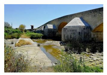
Figure 4. The bridge during the dry season, when the paving blocks of the roman *platea* and the concrete boardwalk built in the first half of the 20th century are visible.
