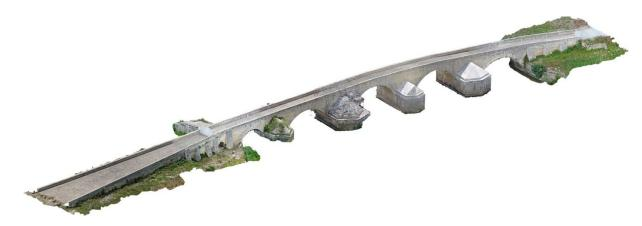
Figure 6. Axonometric view of the bridge elaborated using drone technology and aerial photogrammetry.
