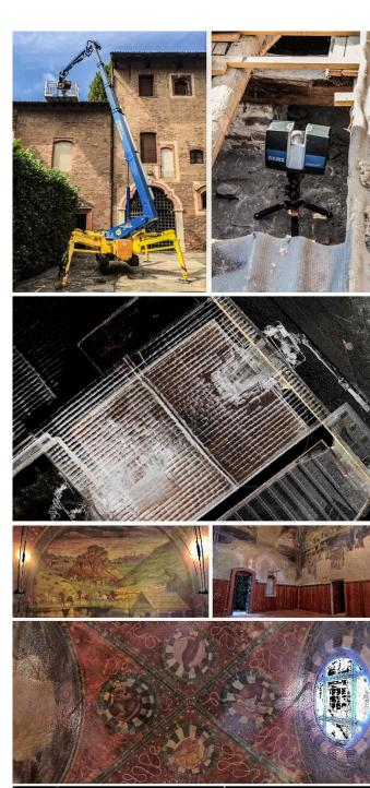
Figure 5. From the top: spiderlift elevator platform used to access the extrados of the chapel vault. Images of the TLS point cloud: in the first one is visible the elevator platform and the dimension of the access to the attic. Image below: Slice of the point cloud. It is one of the control points used to check the thickness of the vault. In the upper part of the image (white/grey profile) are visible the profiles of the bricks.
