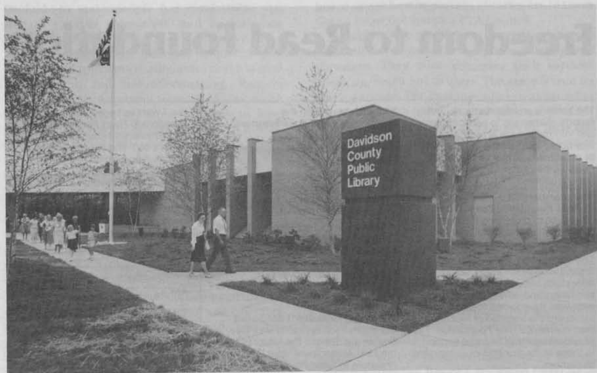
The new Davidson County Public Library is a renovated grocery store.
