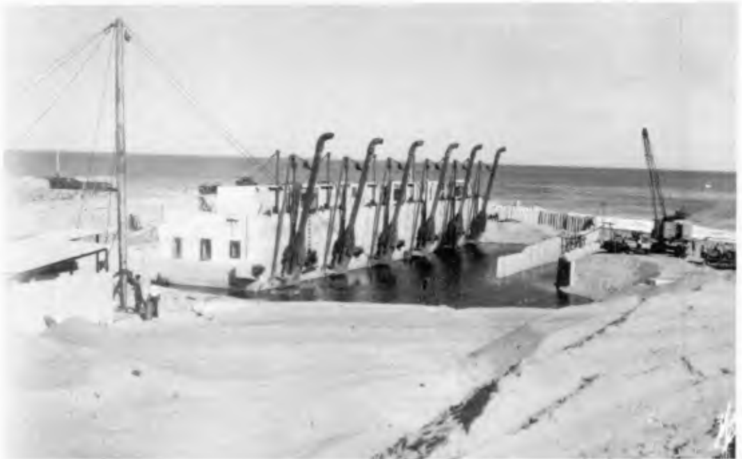
Fig. 3 Preliminary arrangement to control moving sand
