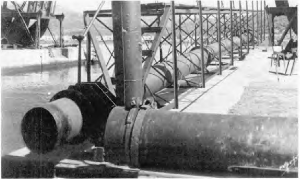
Fig. 4 Half section of swing bridge across the entrance to the basin, in open position.
