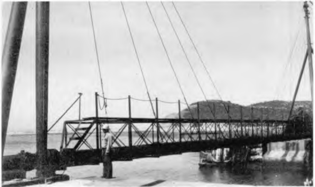
Fig. 5 Complete swing bridge in closed position.
