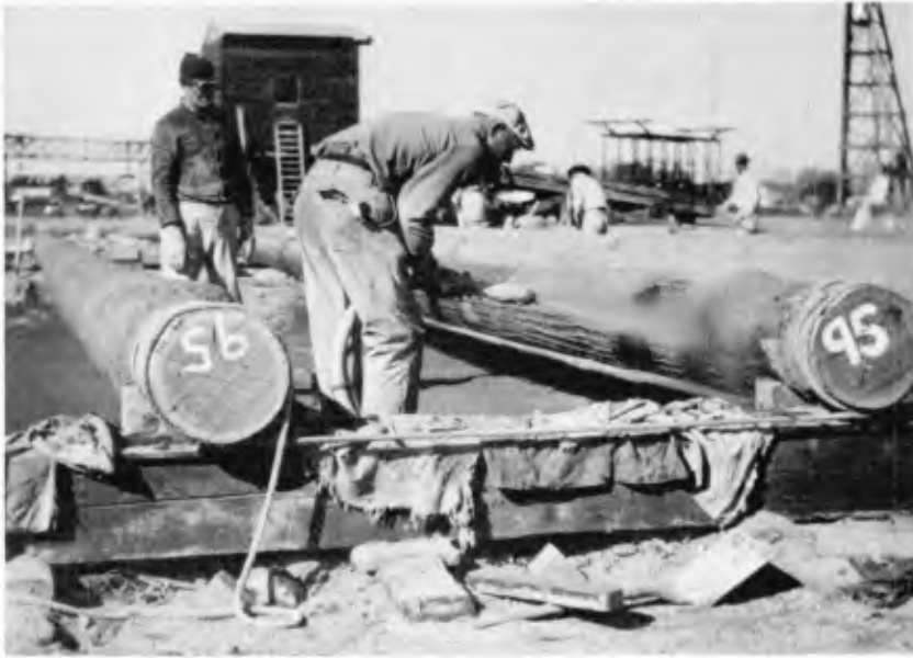
Fig. 7. Gumite being placed on wood pile.
